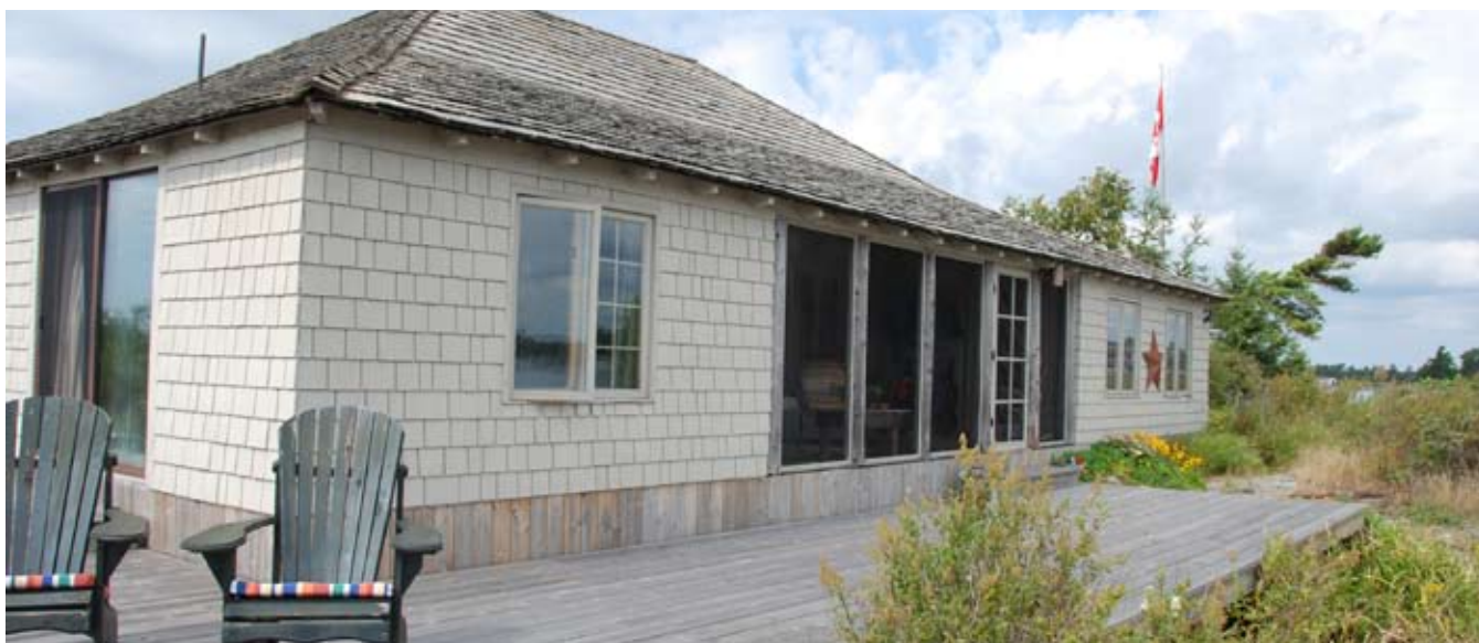
Screened-in Porch/Wrap around deck
